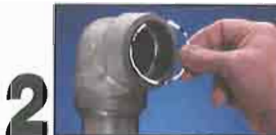
2 Fitter seats ring into fitting. Spring tension holds ring lightly in place, assuring no rattling or vibration even under extreme pressure. Ring actually becomes a permanent part of the joint.
