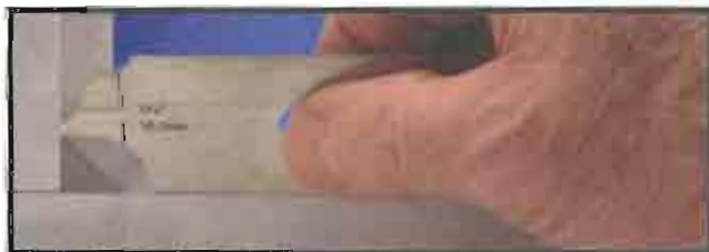
CHECKING FILLET LEG SIZE
