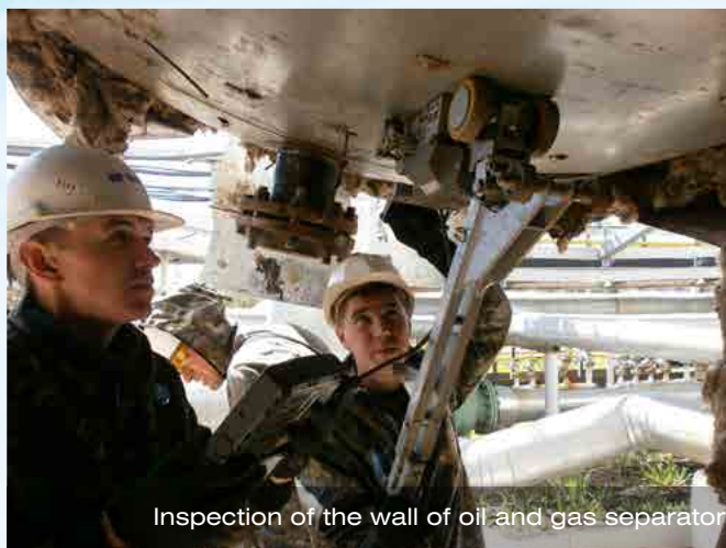
Inspection of bottom level of tank wall
